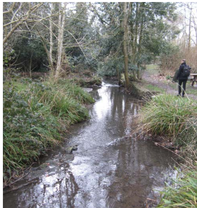
Vegetation beginning to break up wall structures
